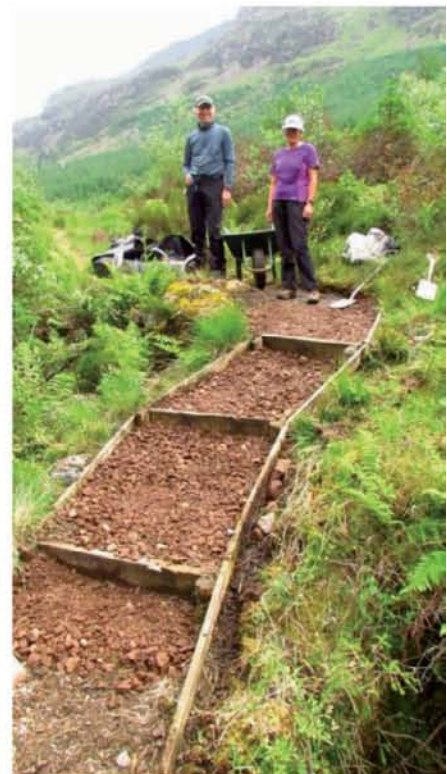
Volunteers repairing the Liza Path.
