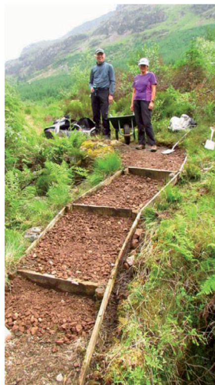
Volunteers repairing the Liza Path.
